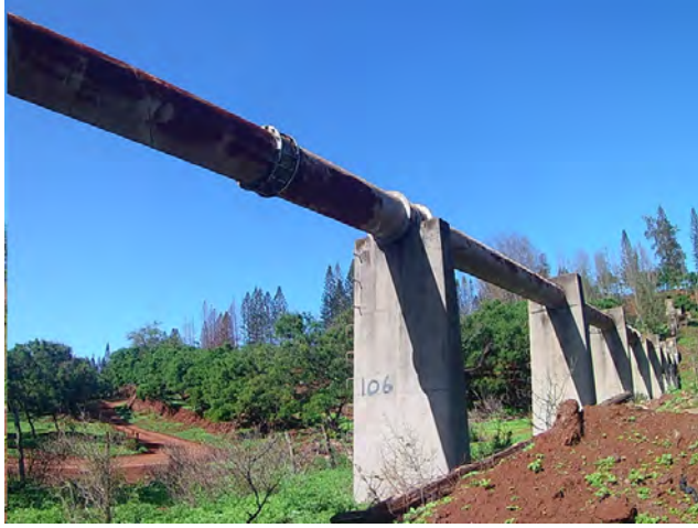
Coupling 106 (north side)
