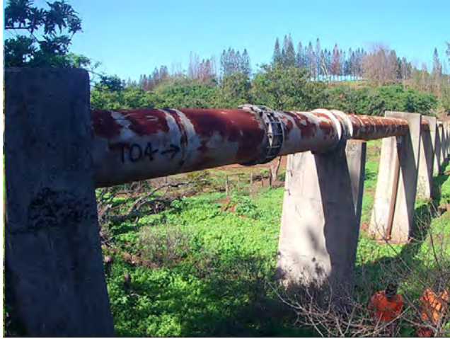
Coupling 104 (north side)
