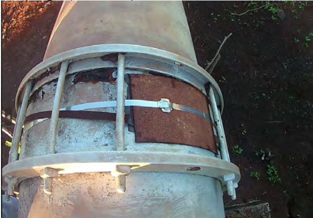
Coupling 1 (north side)
